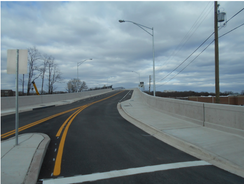
Picture Below: Bridge – Looking North from the Roundabout
