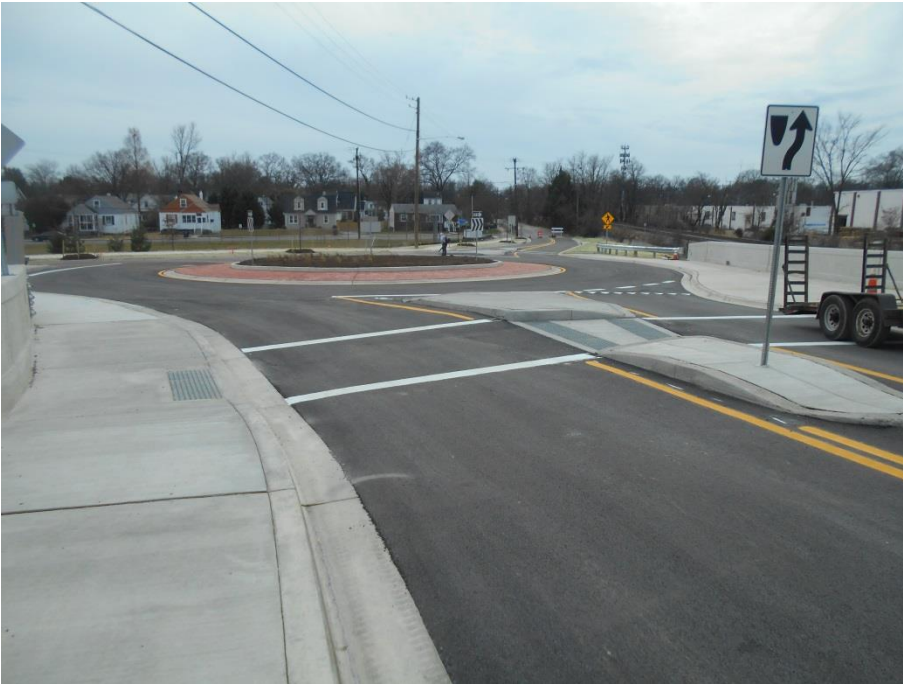
Picture Below: Roundabout at Rivertech Court Extension
