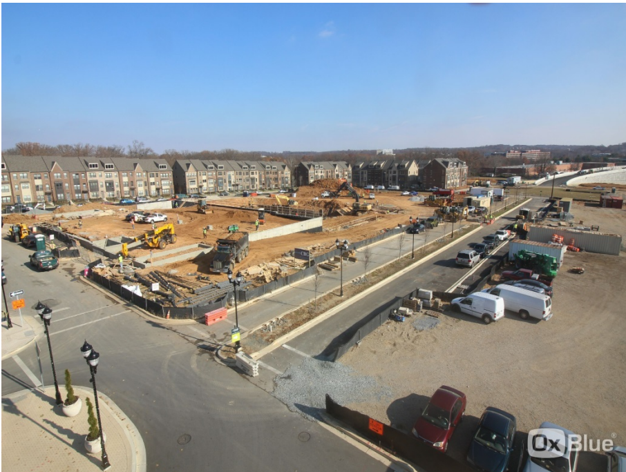
Picture Below: Building 5 parking garage
