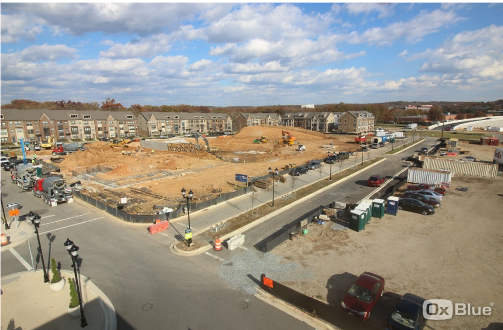
Picture Below: Parking Structure Progress on Parcel E – Building 5 Site
