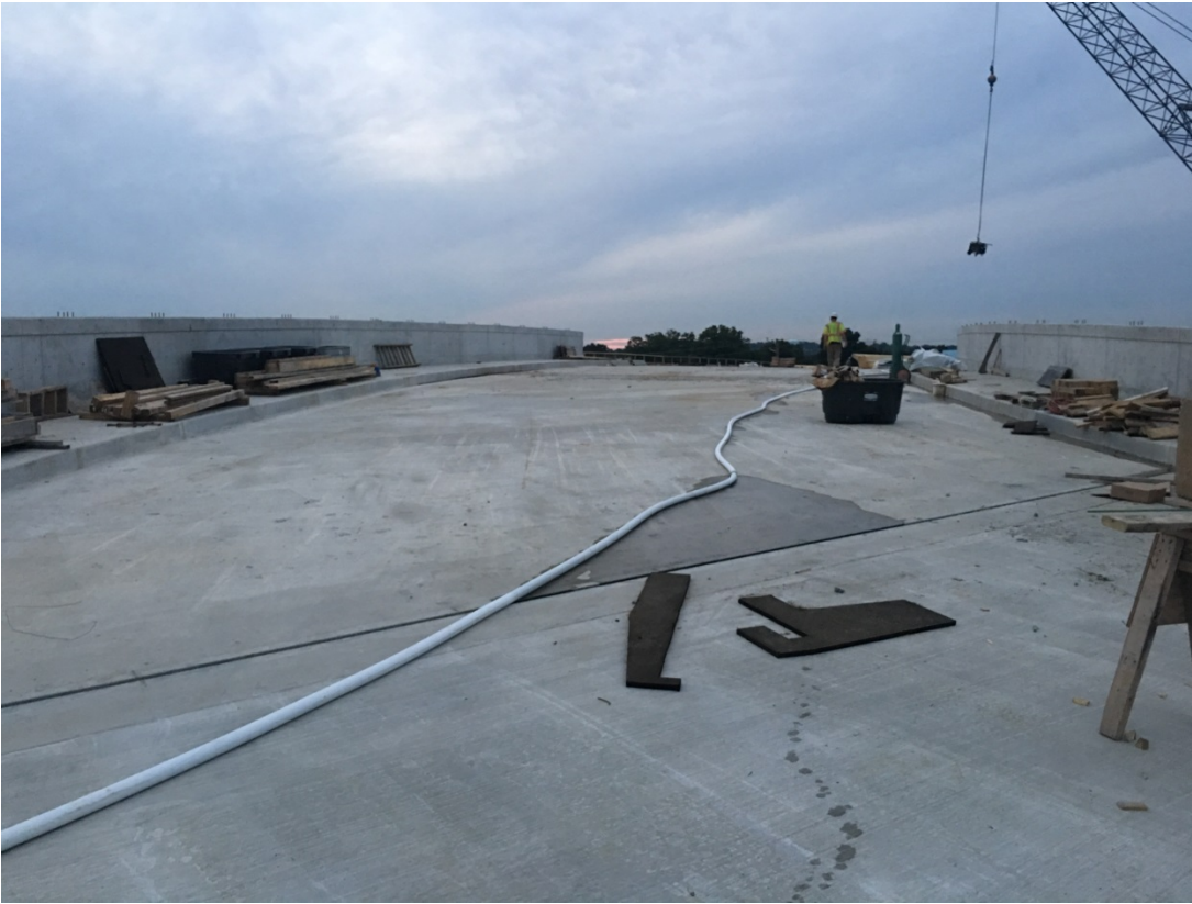
Picture Below: Bridge Deck – Looking East
