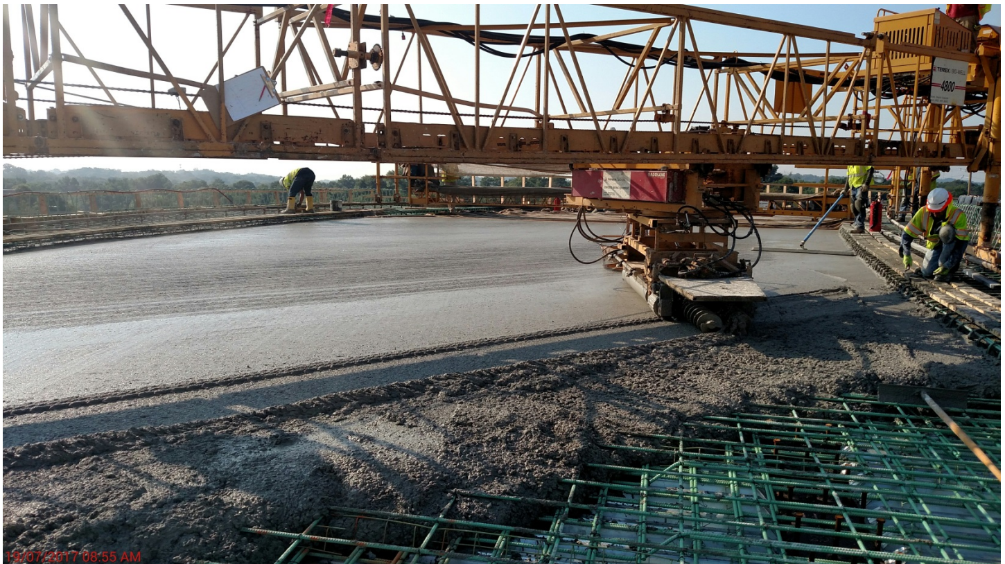
Picture: Bridge Deck – July 19, 2017
