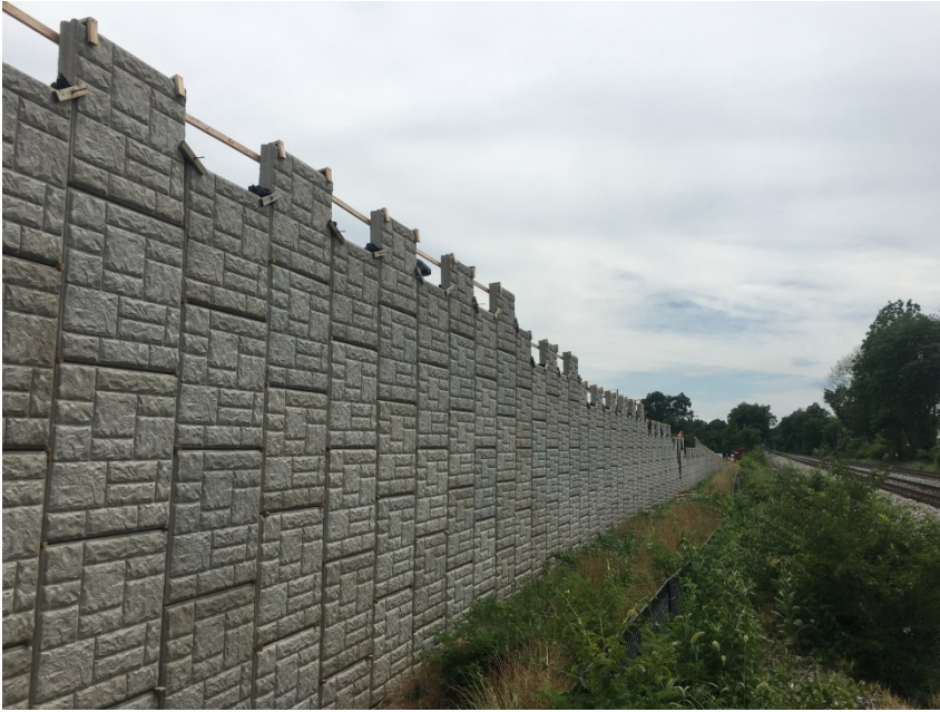
Picture: Bridge MSE Wall along CSX Tracks – Looking South: July 2017
