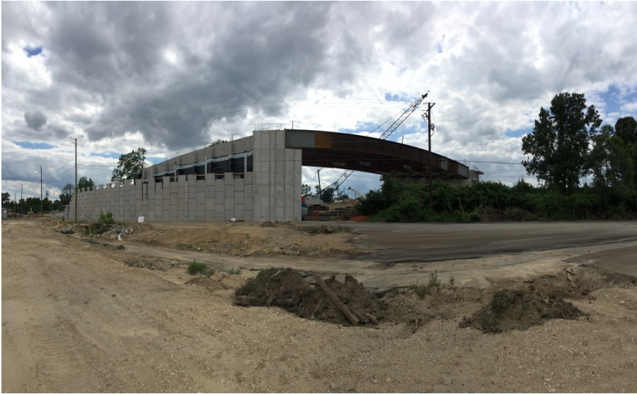
Picture: CSX Crossing – from the west looking north: June 2017
